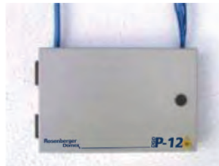
DGO P-12 attached to wall, entrance of optical cable and cord outlet
