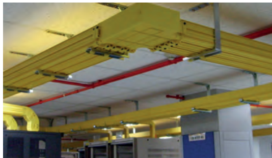
Infrastructure installation, treadmill - Raceway conduits
