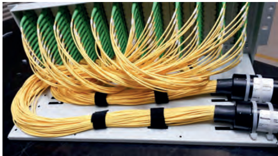
Cable installation - Trunk
