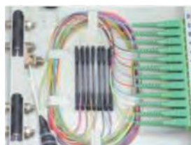
Fitting of splicin pigtaills
