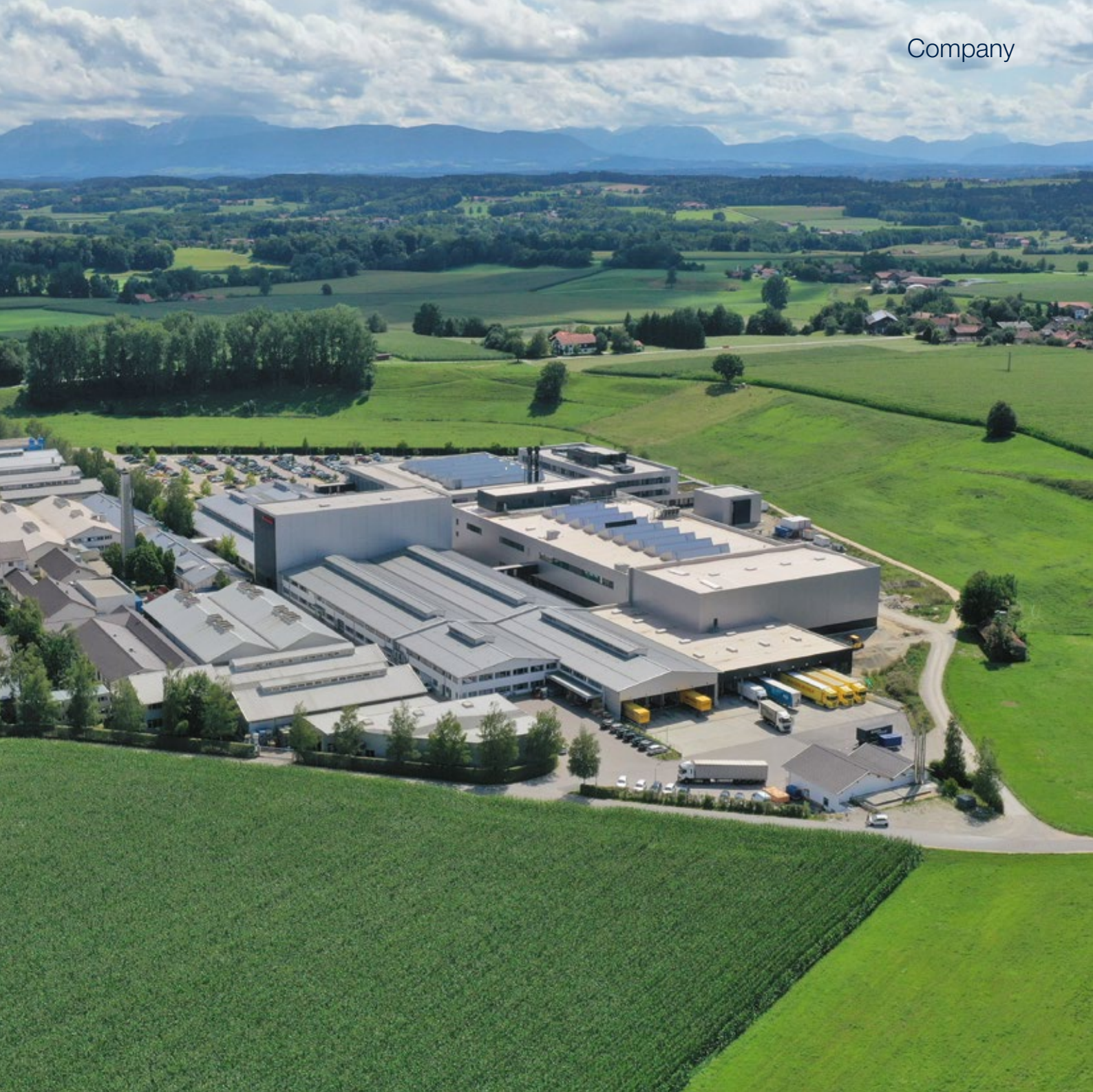
The Rosenberg headquarters located in Fridolfing in the southeast part of Bavaria, Germany
